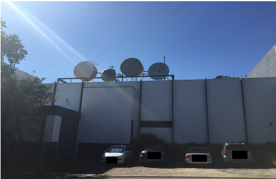
Photo 2: Looking east across the site with communications infrastructure visible on the roof
