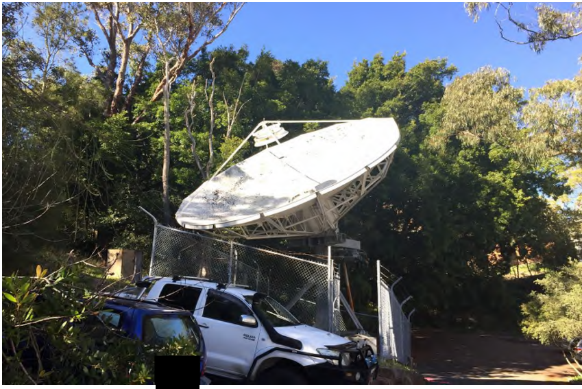
Photo 10: Satellite dish (disused) on the eastern portion of the property
