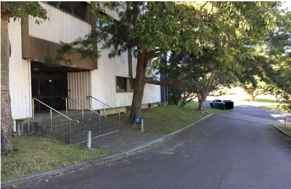
Photo 6: Asphalt surface condition along internal roadway
