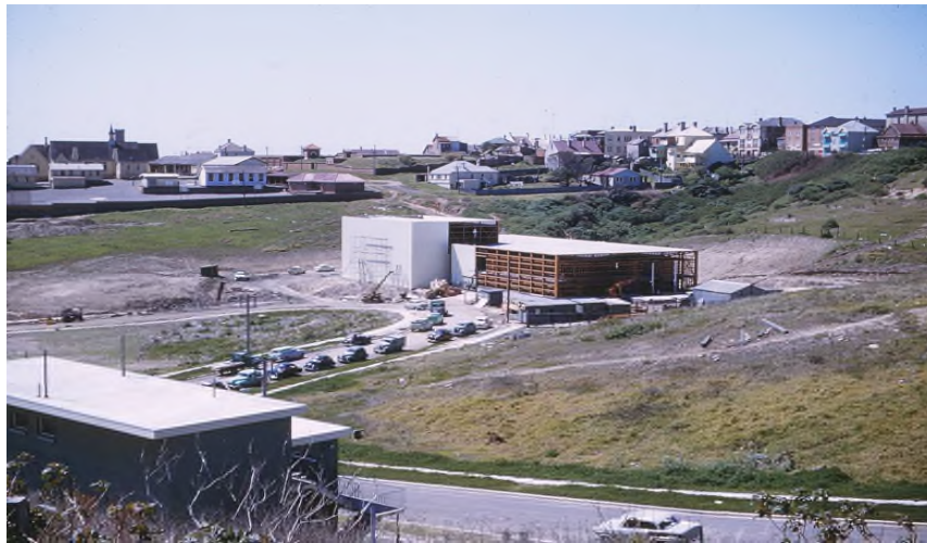
Photo 12: Historic image of progression of construction taking place into the cut in the hill. Photo Credit (Unknown) - Sourced Newcastle Lost Facebook Page (September 2018)
